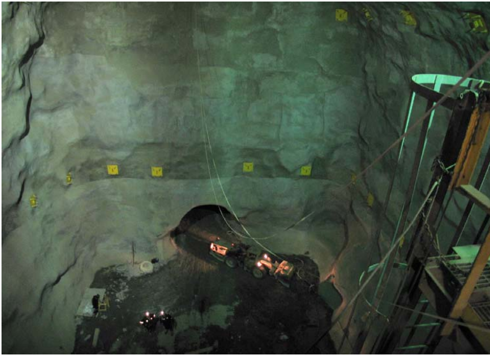
Illustration 1: Looking down into the Cube Hall.
